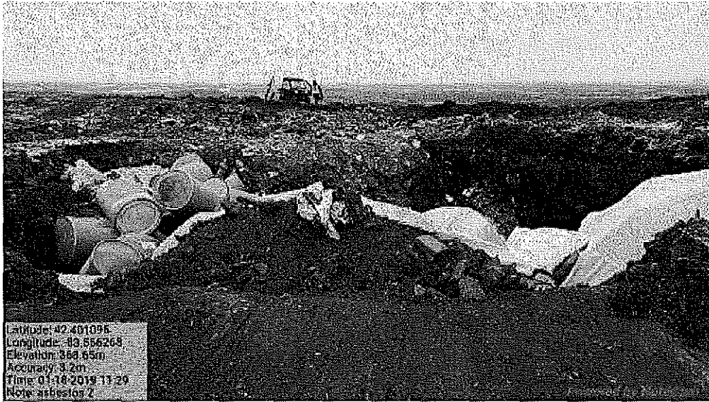
Image 10(Asbestos Disposal) : Asbestos Disposal
