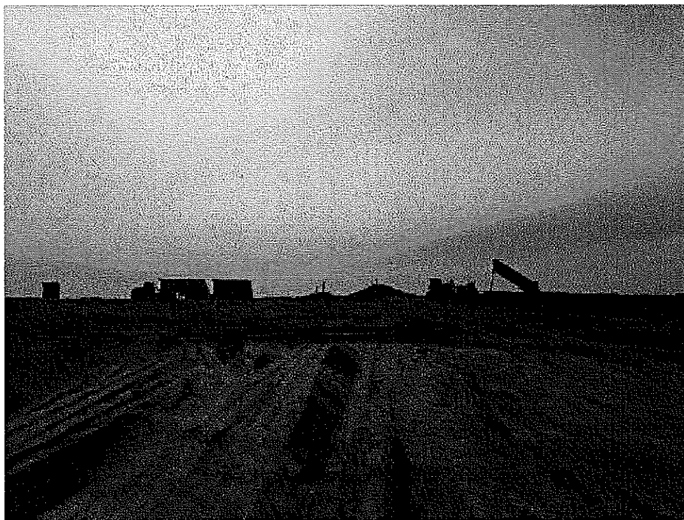
Image 1(Top of landfill) : New grading of top of landfill.
