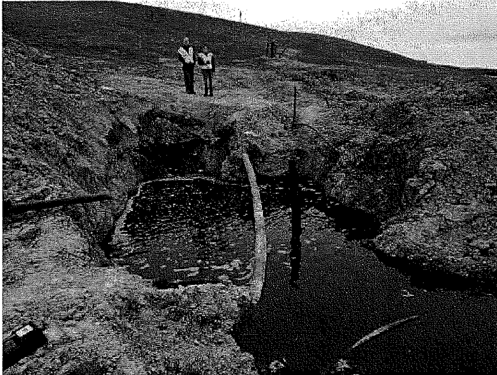
Image 5(New Leachate Break) : Horizontal well leachate breakout 200 yards West of TS-01.
