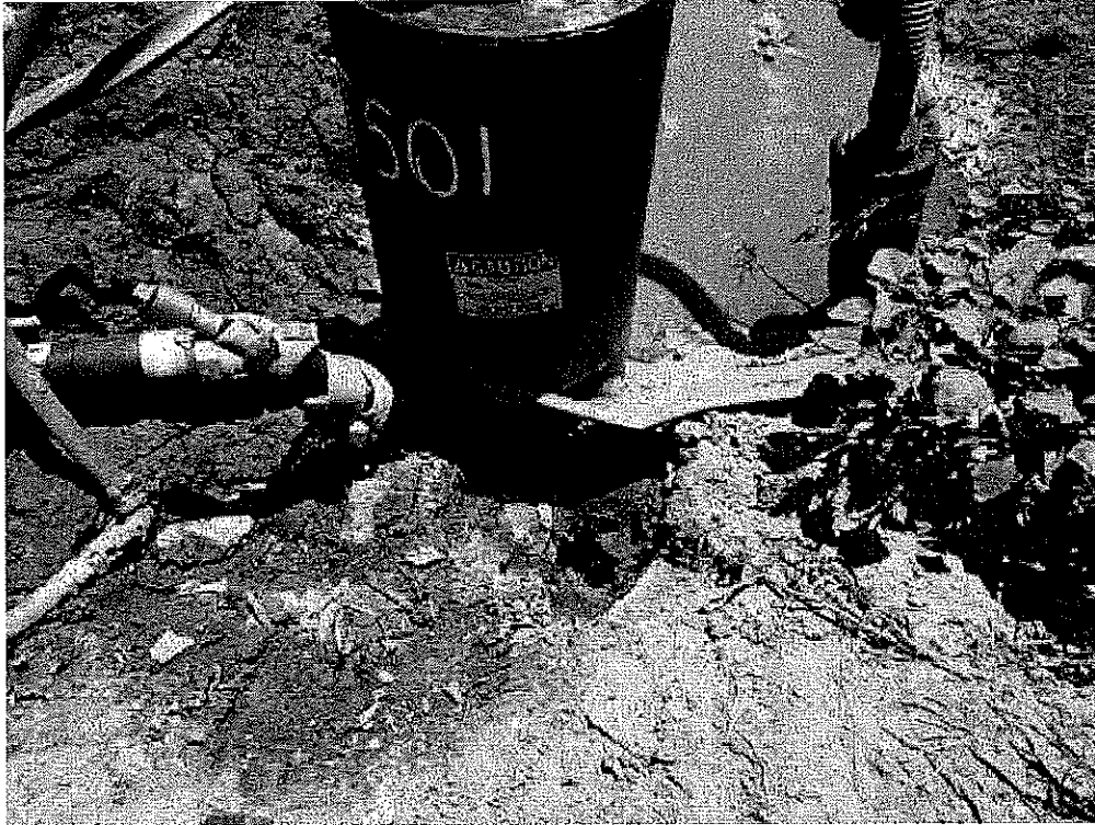
Image 1(TS-01 Gas hole) : TS-01. Note gas hole at base.
