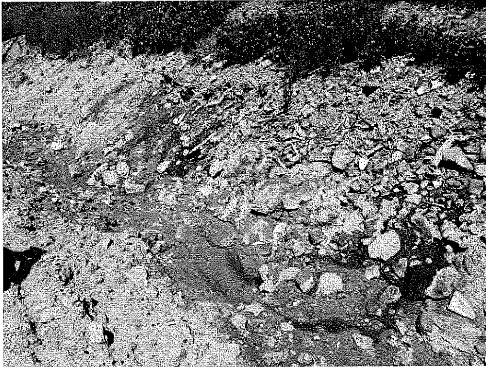
Image 3(Small leachate seep) : Small leachate seep along West haul road ditch.
