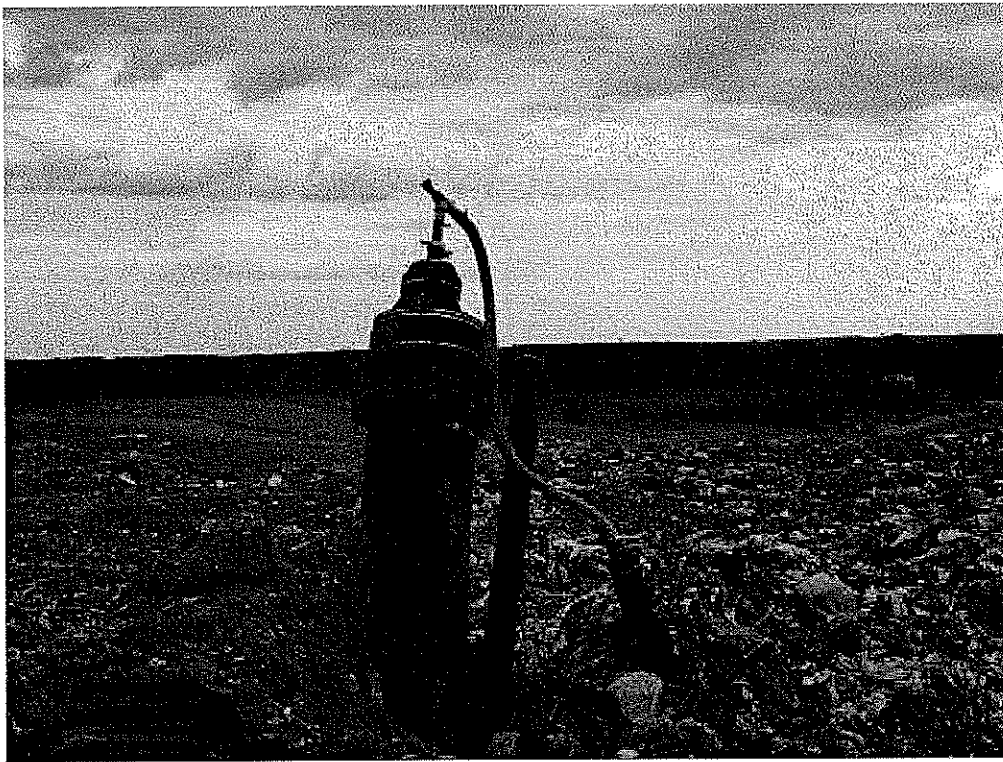
Image 3(Well head N side.) : Well head North side.
