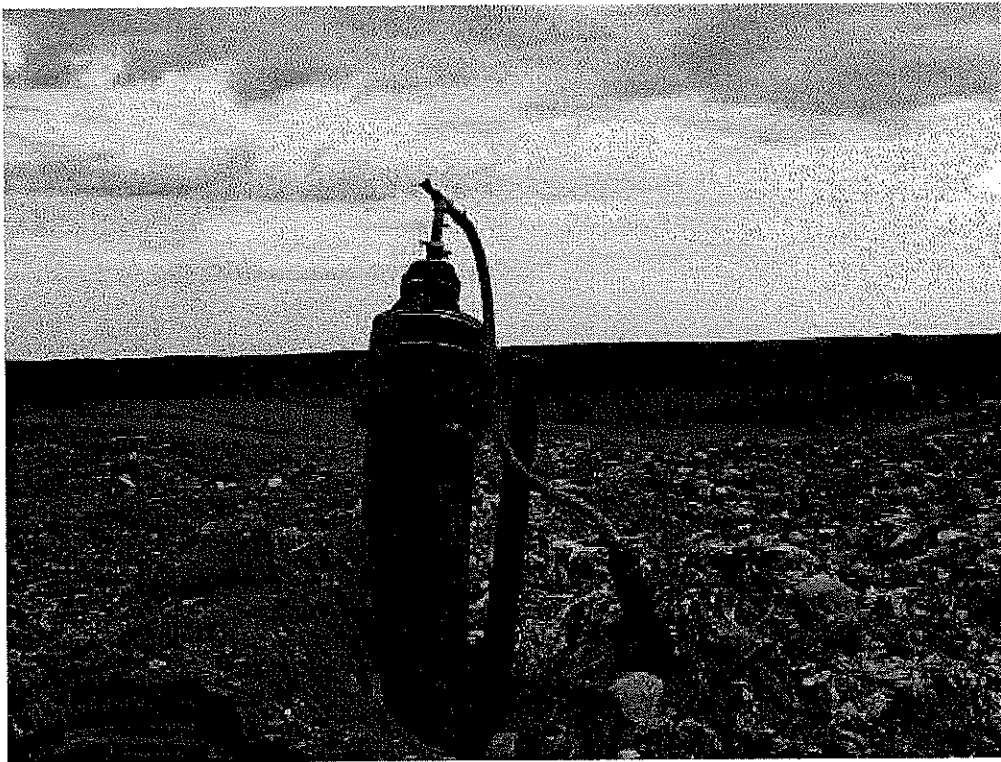
Image 4 (Range 6 Wellhead) : Area beyond North side.
