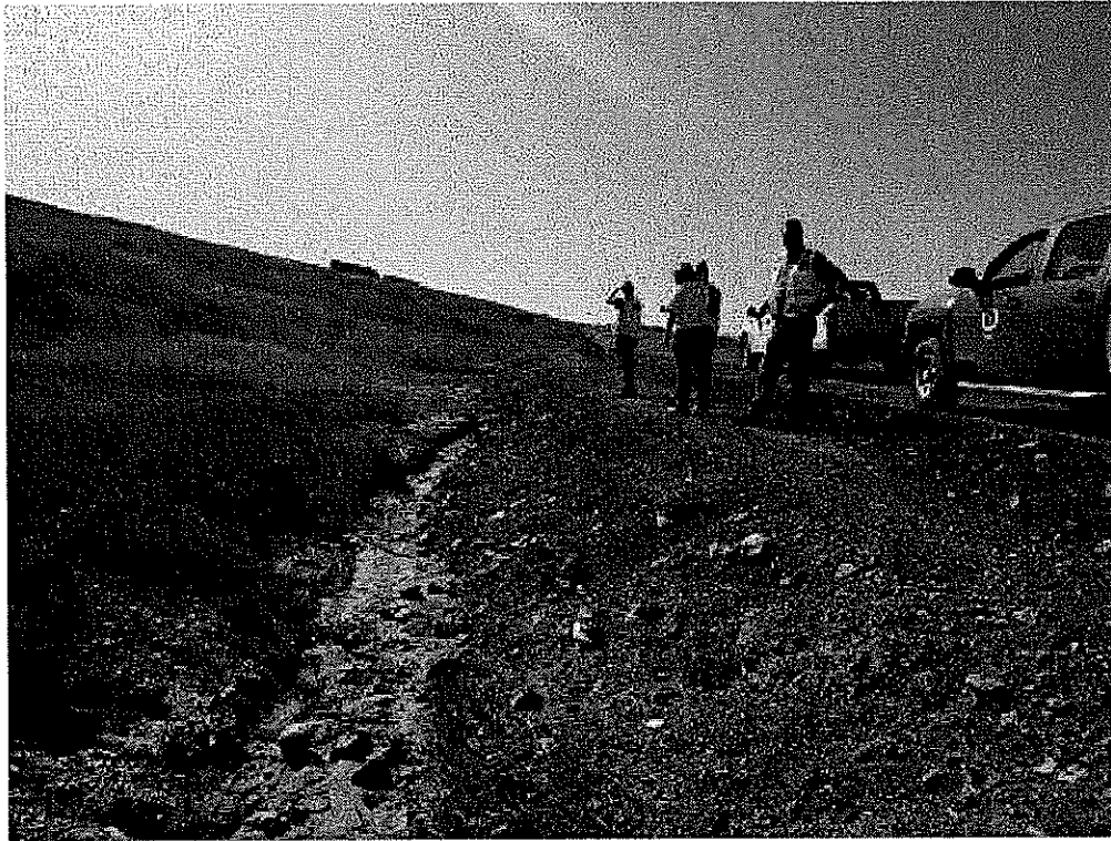
Image 6(Well haul road ditch) : Well haul road ditch.
