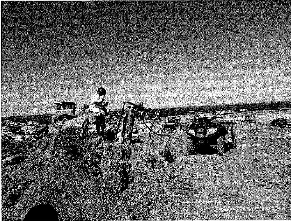
Image 8(Down hole testing) : Down hole testing.
