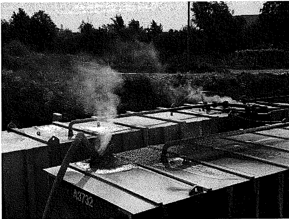
Image 7(Frac tanks) : Frac tank emissions.
