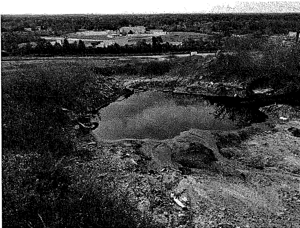
Image 9(TS-01 pond) : TS-01 pond that is being removed.
