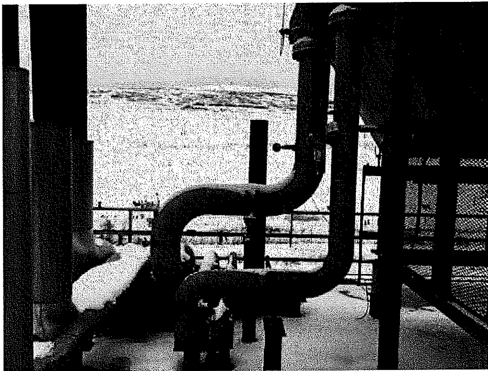
Image 2(Compressor Vent) : One of four compressor vent stacks.
