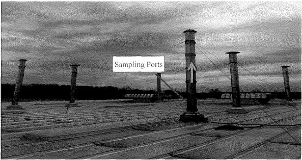
Figure 2-5 Post Quench Washer Sampling Location
