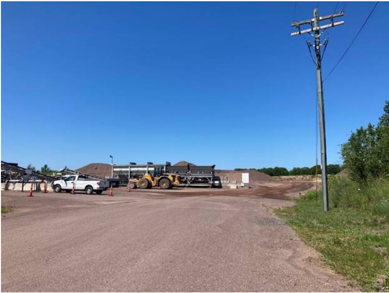
Image (1): Plant roadways
