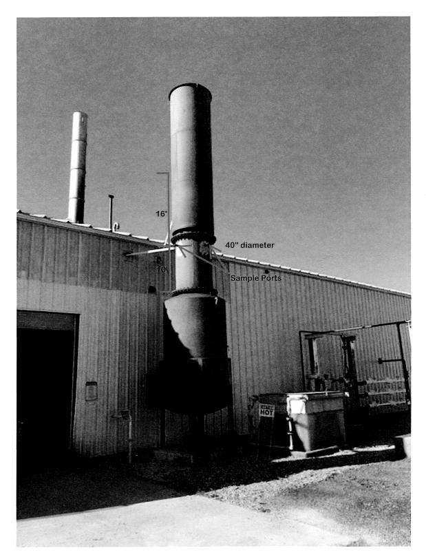
**Representative Photo – Turbine Exhaust Stack** Diagram for EUTUR01-EUTUR02
