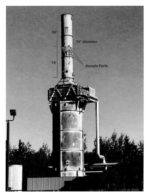
**Representative Photo - Heat Media Heater** Diagram for EUPLANT2HEATER-EUPLANT5HEATER
