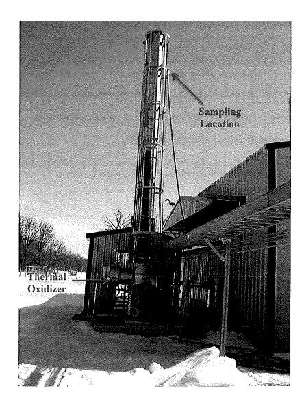
Figure 2-3. Eaton Rapids Thermal Oxidizer Exhaust Stack
