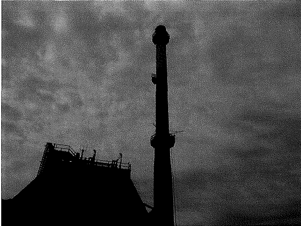
Image 1(GPS Boiler Stack) : Testing setup on stack
