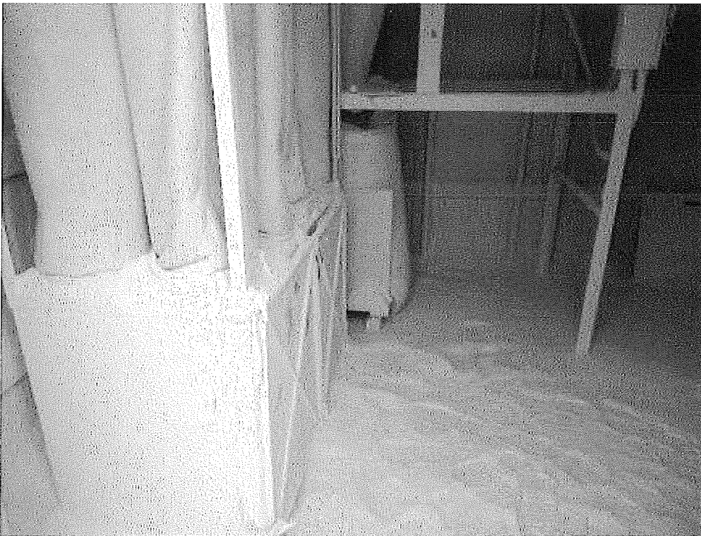
Image 2(Dust Room) : Looking to the south inside the Dust Room.
