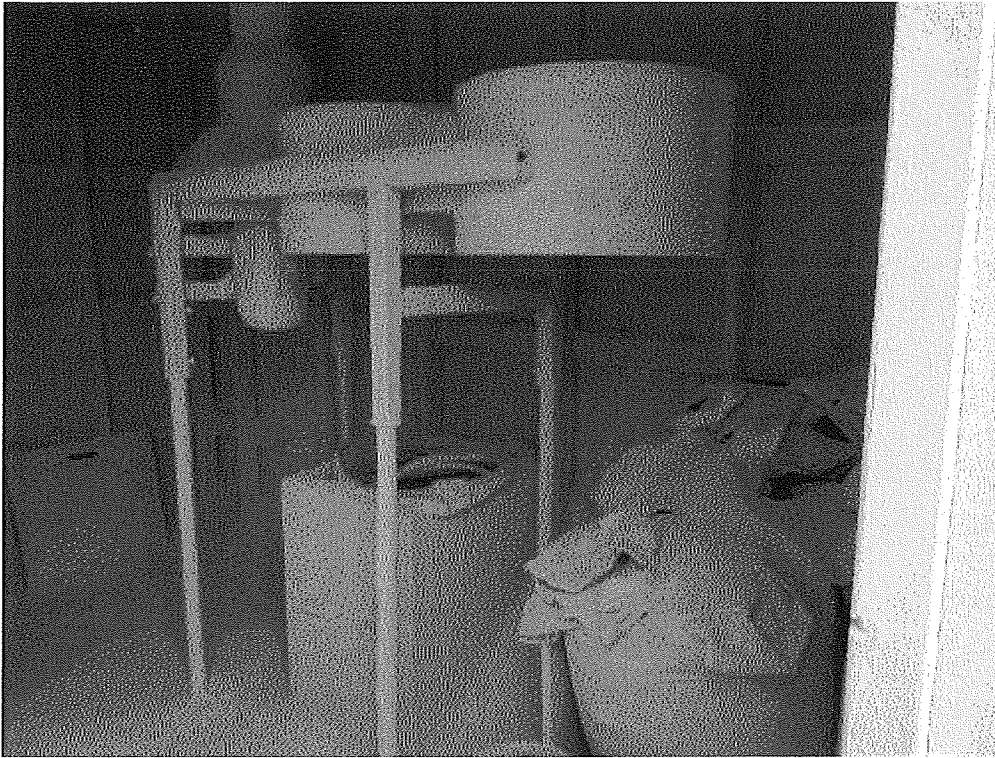
Image 4(Dust Room) : Looking to the north inside the Dust Room.
