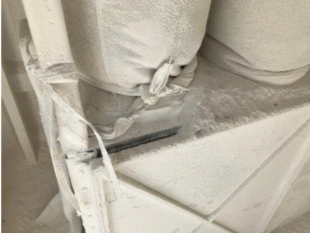
Image 4(Baghouse 4) : Image shows where collection bin seal is failing to contain particulate matter.
