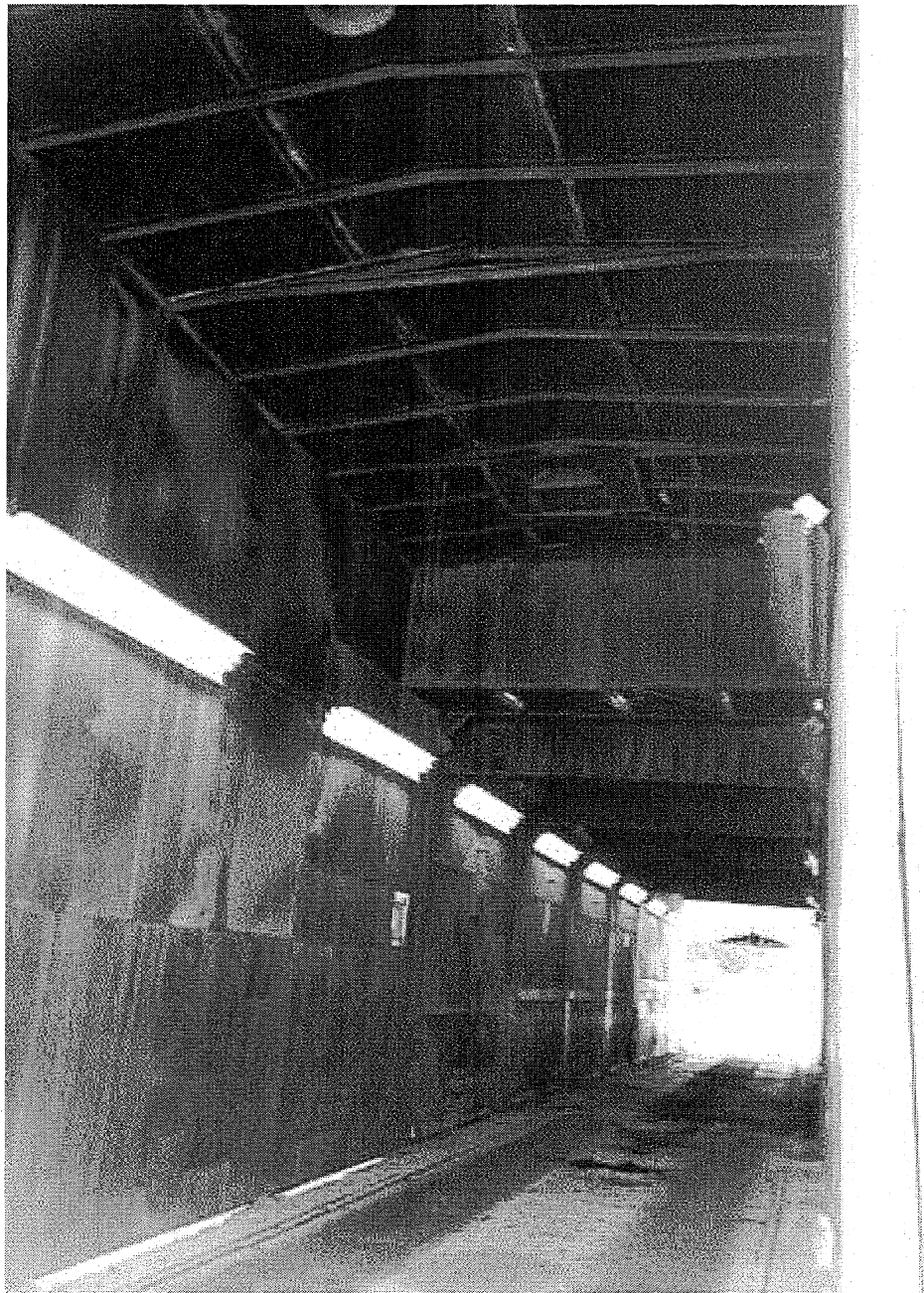
Image 10(Figure 10) : Interior of the loadout enclosure, 8/22/15, 10:20 am.
