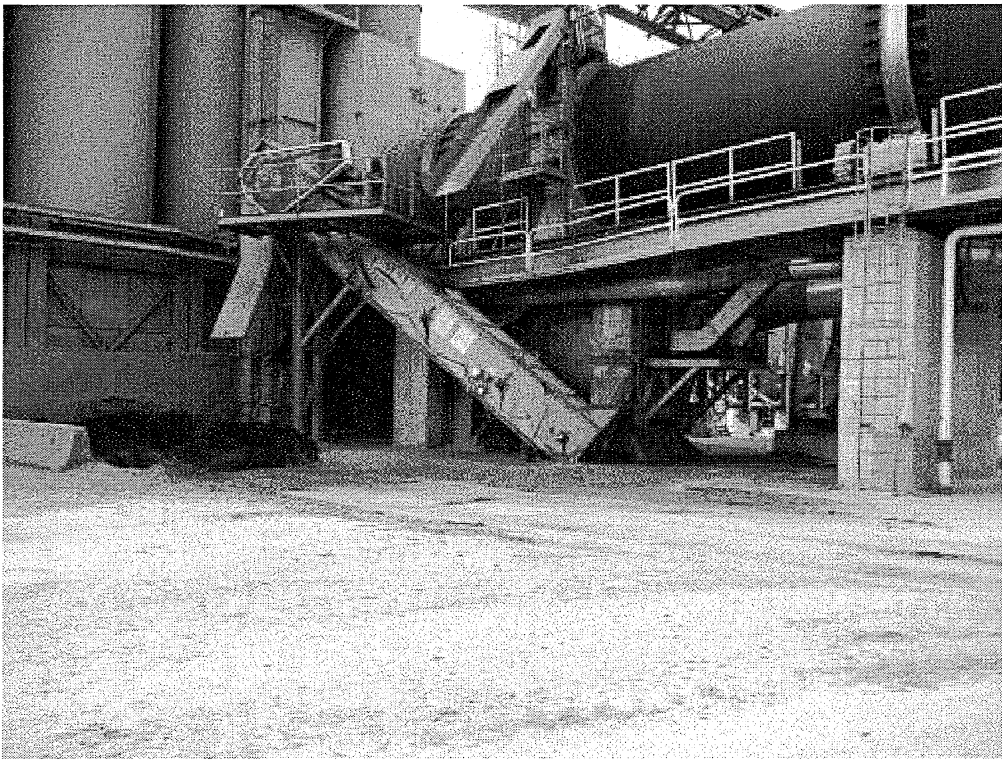
Image 5(Figure 5) : The dual drum dryer and mixer, 8/22/15, 10:15 am.
