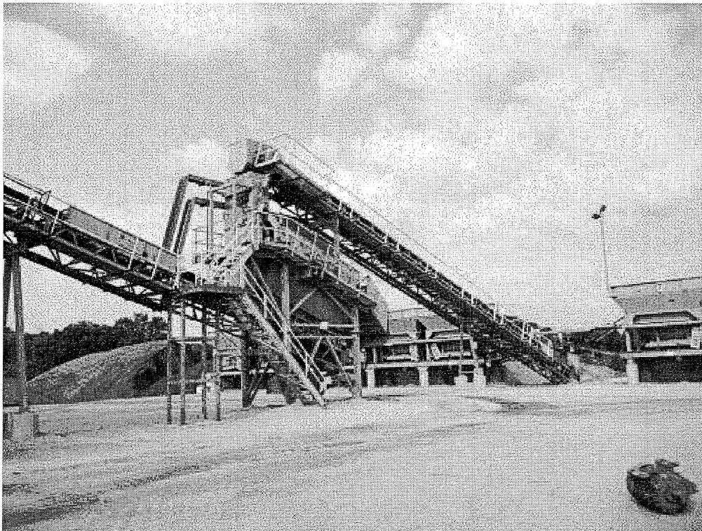
Image 3(Figure 3) : The aggregate conveyers, 8/28/15, 10:15 am.
