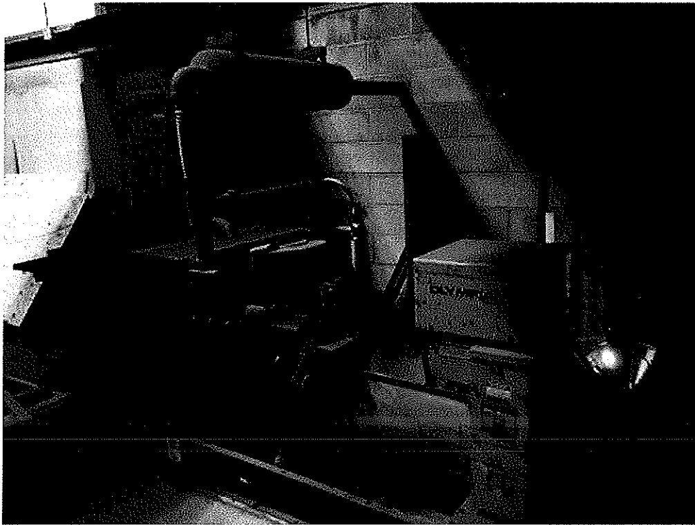
Image 6(0021) : Natural gas-fired generator set
