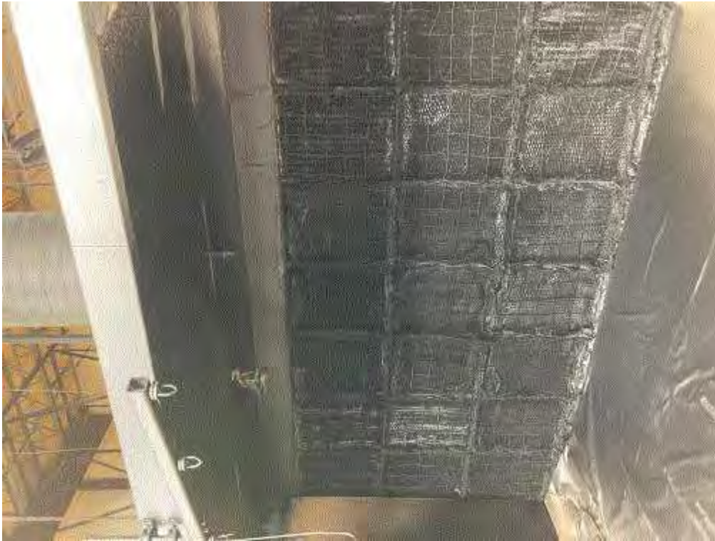
Image 3(IMG_0121) : Spray booth for application antiquing finish
