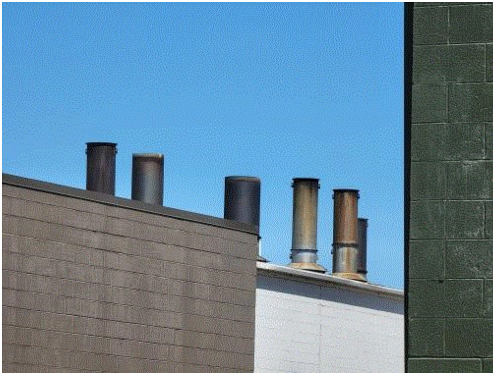
Image 1(20220513 115248.jpg) : View of exhaust stacks at 4900 Fernlee from 4815 Delemere Avenue. From left to right, the stacks are aligned from south to north. At this location, the view of the north most stack is partly obstructed by the adjacent stack.
