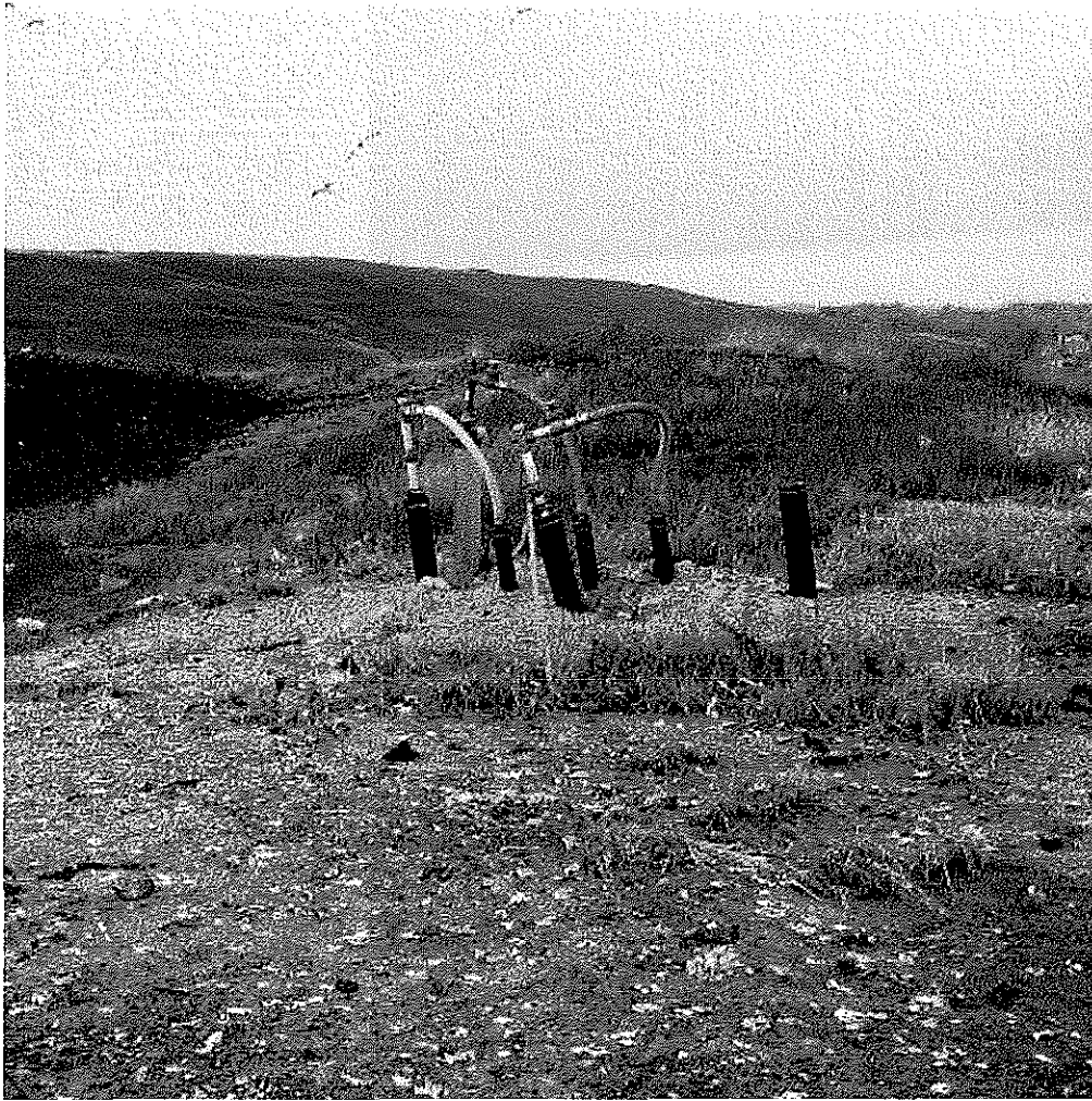
Image 3(Gas wells) : LFG wells near the active face of the landfill.
