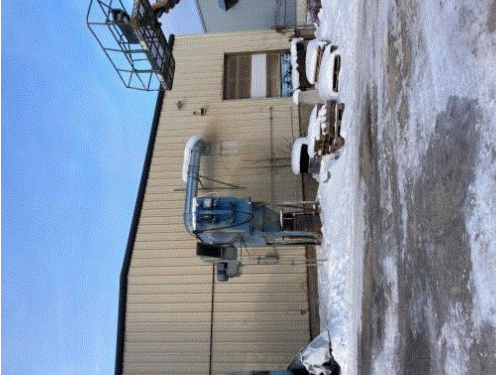
Image 1(EUSANDBLAST) : Cartridge filter collector for sandblasting operation.
