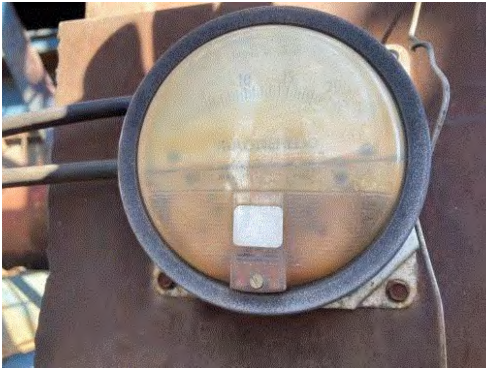
Image 2(2) : Inoperable pressure drop gauge for cyclone and/or wet scrubber.
