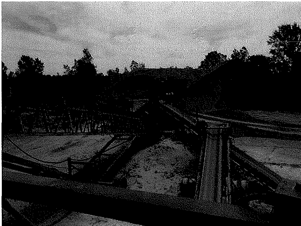
Image 3(Plant view) : Feeder, conveyors to crusher
