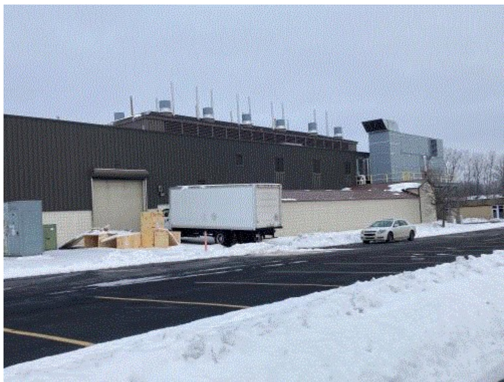
Image 1(Building/Roof stacks) : Building/Roof stacks.
