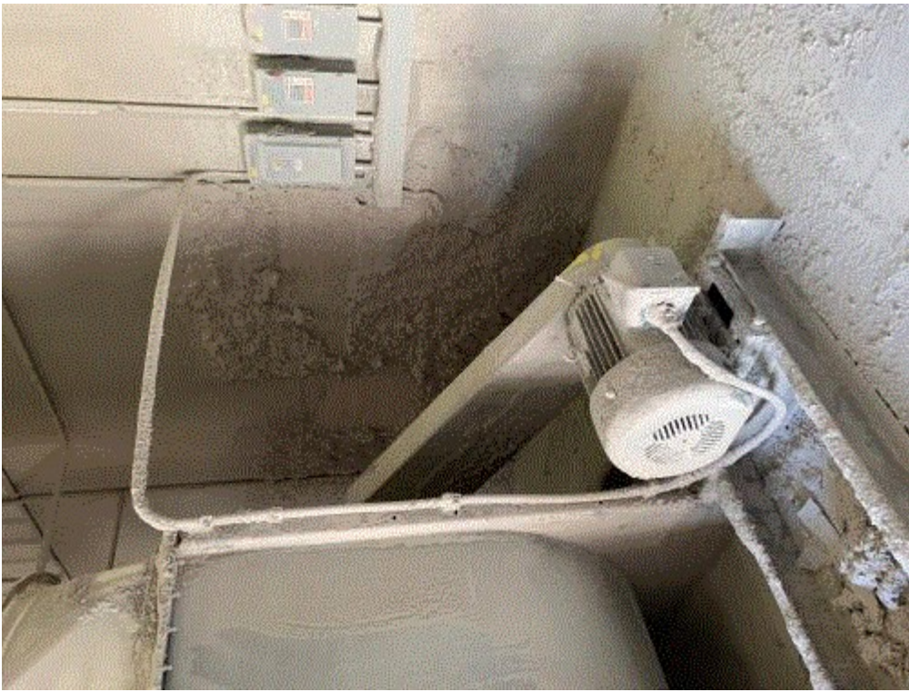
Image 2(Nu-Wool) : General baghouse room conditions (accumulation of material on the walls)
