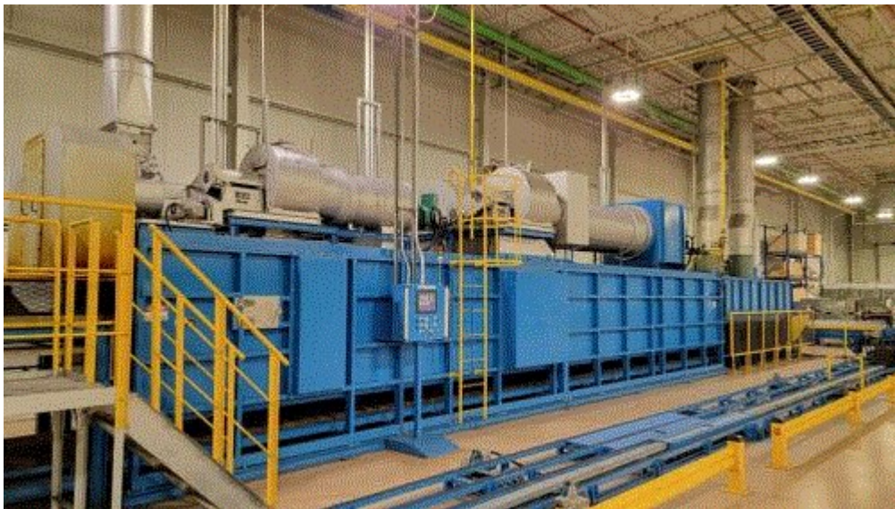
Image 1(Coating Line) : Dip/spin coating line that uses low VOC coatings.
