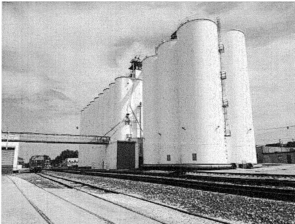
Image 6(New storage silos) : New storage silos associated with grain elevator.
