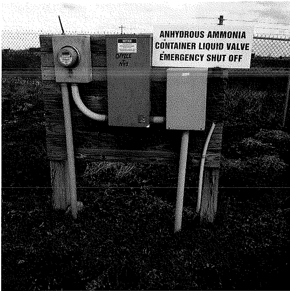
Image 4(008) : Remote emergency shut off valve
