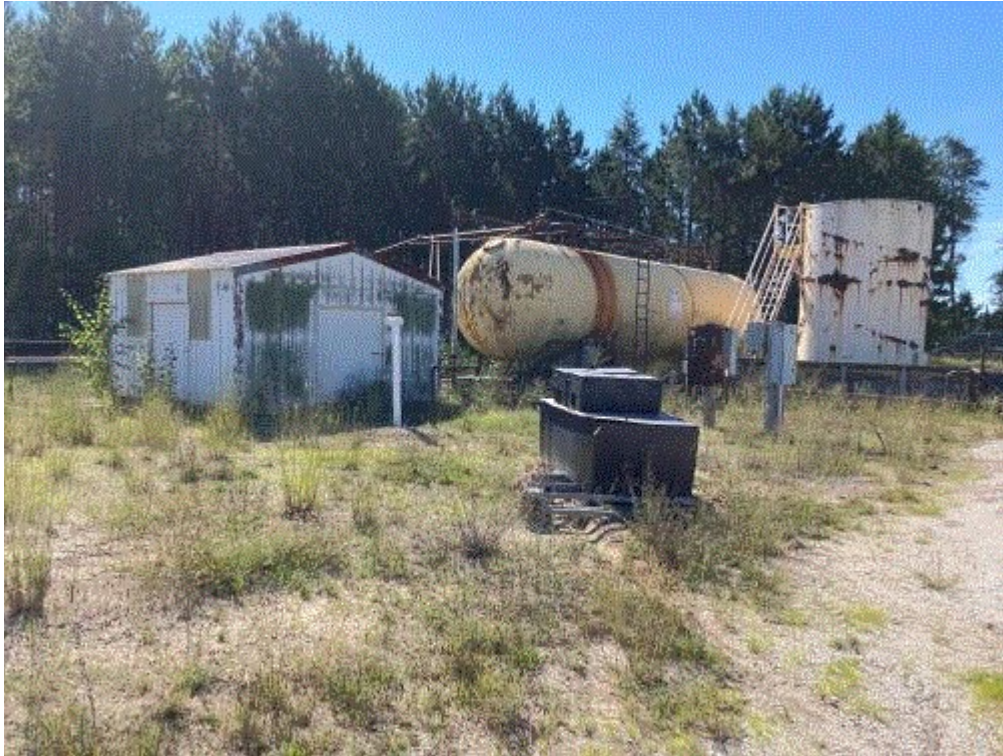
Image 5(Tanks & VRU) : Tank Battery and VRU building
