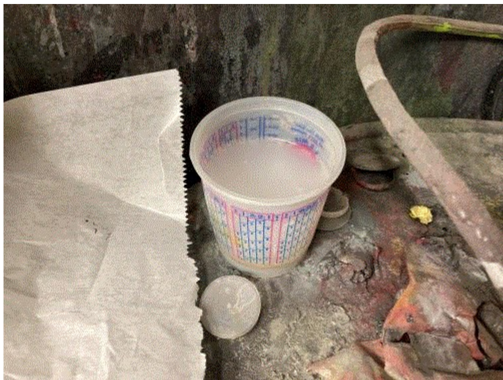
Image 7(IMG_0221.JPG) : May 14, 2021, open cup of solvent in the paint mixing room.
