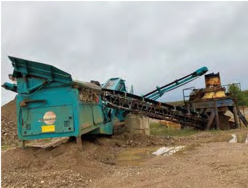
Image 1(1) : Crushing plant GPTI 187-08
