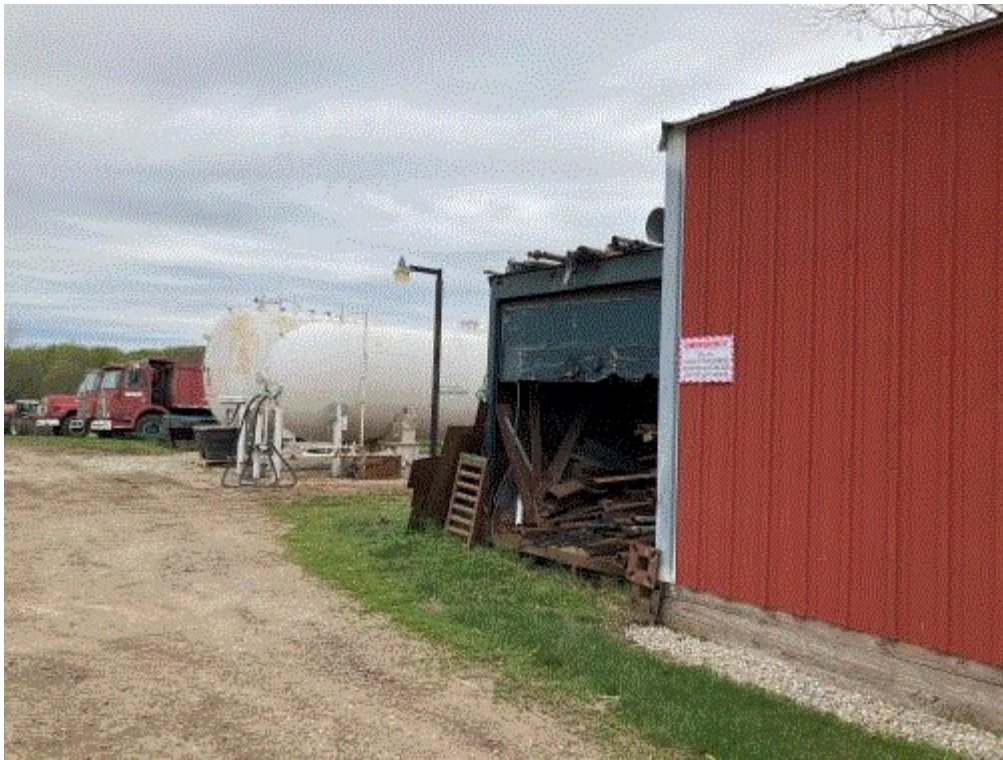
Image 4(Contact sign) : Emergency contact sign located on red barn, south of the anhydrous ammonia tank.
