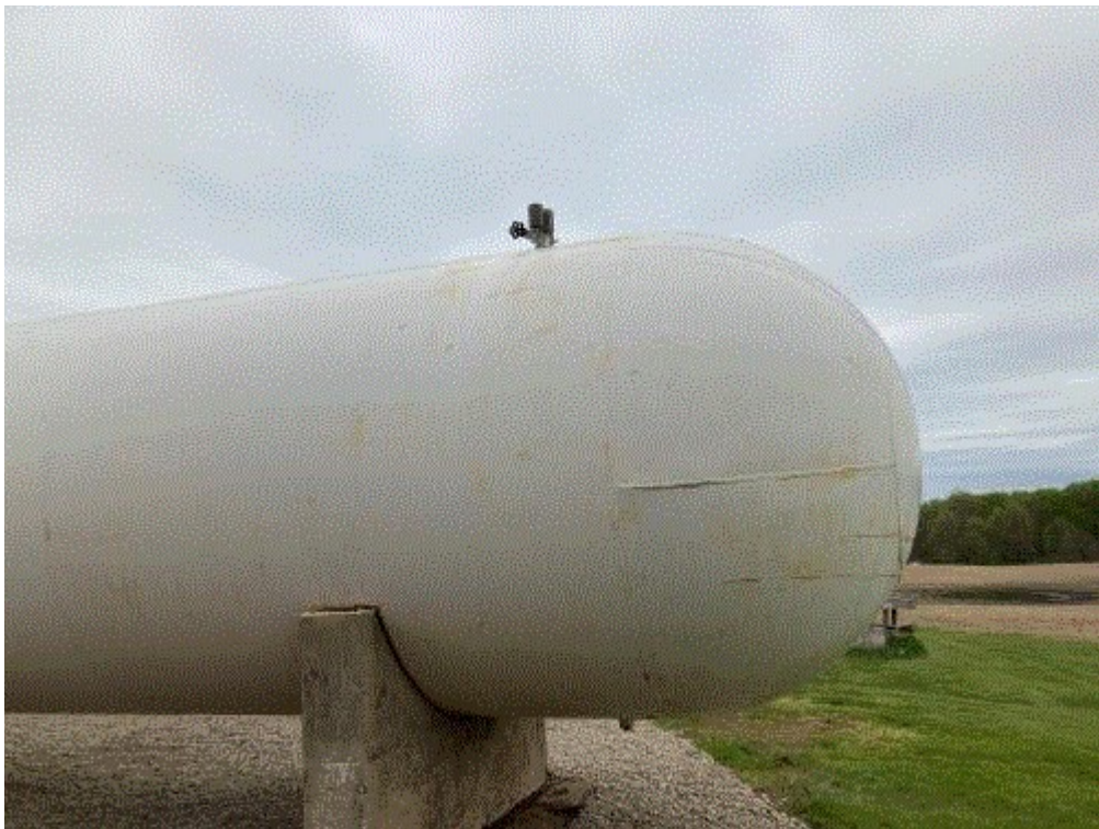
Image 7(Safety Relief Valves) : Safety Relief "pop-off" valves located on top of tank to the rear.
