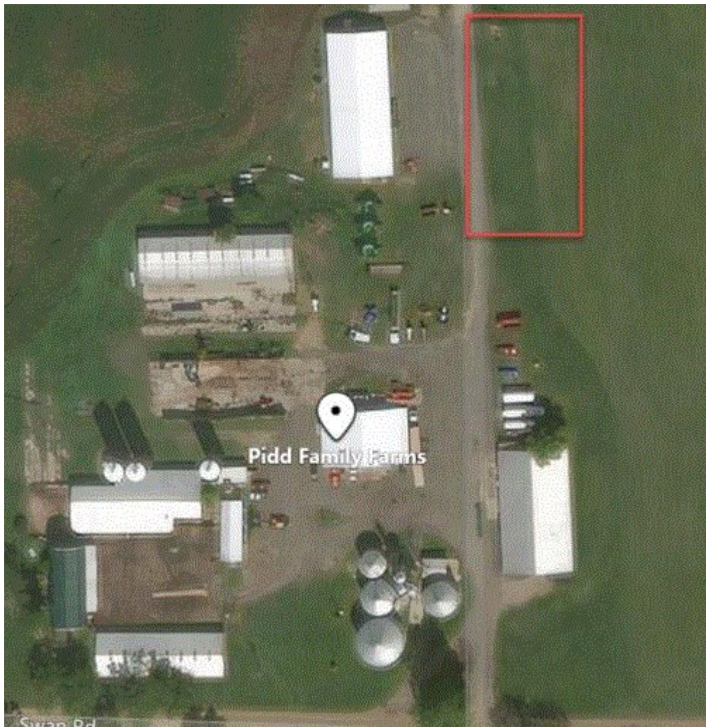
Image 3(Nurse Tank Location) : Red square indicates the general location of where the anhydrous ammonia nurse tanks and applicator tank are stored.
