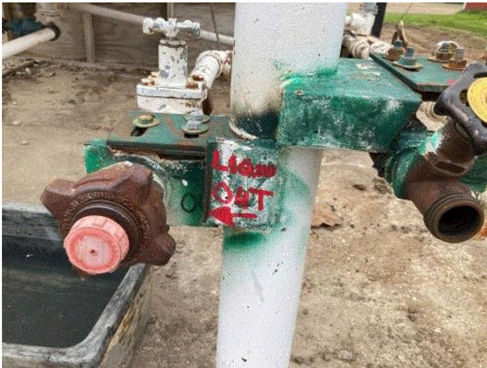
Image 12(Bulkhead Mods) : Modifications to bulkhead to ensure that, for example, the "Liquid Out" line was
