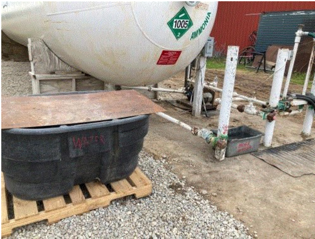
Image 11(Emergency water tub) : T. Pidd moved this tub to a location further away than the location pictured here. This was done per my recommendation to ensure, in the event of an emergency, those impacted would be away from the source of the hazard.
