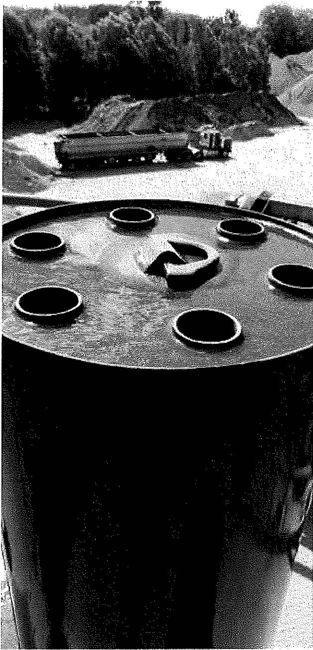
Image 1(Superior Asphalt) : AC Vapor Condensate System
