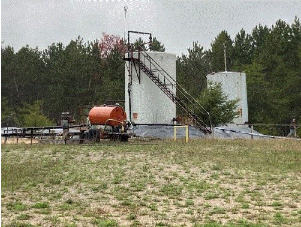
Image 3(spection pic (3-4)) : Northern portion of site, looking at tanks
