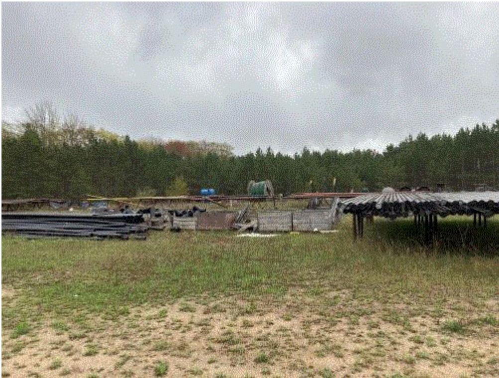
Image 4(Inspection Pic (4-4)) : Eastern storage materials onsite (looking south)
