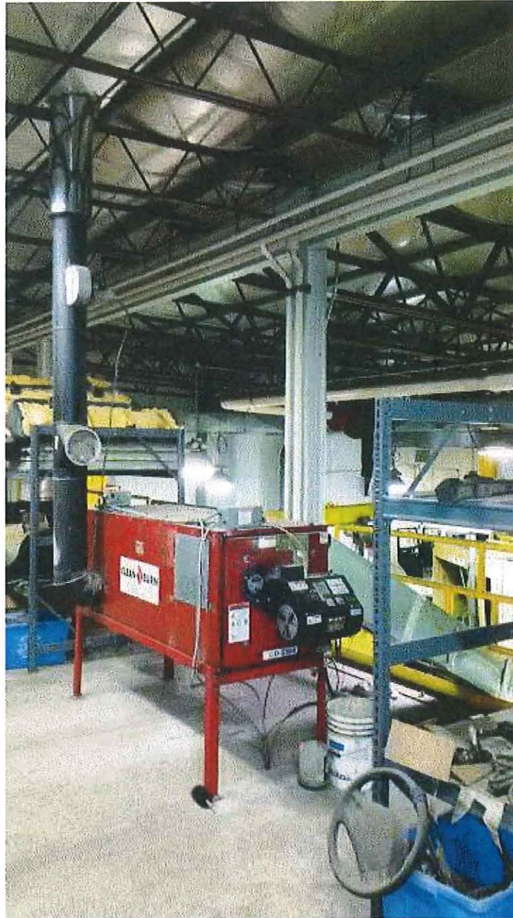
Image 3(CE1) : CB-2500 multi-oil furnace
