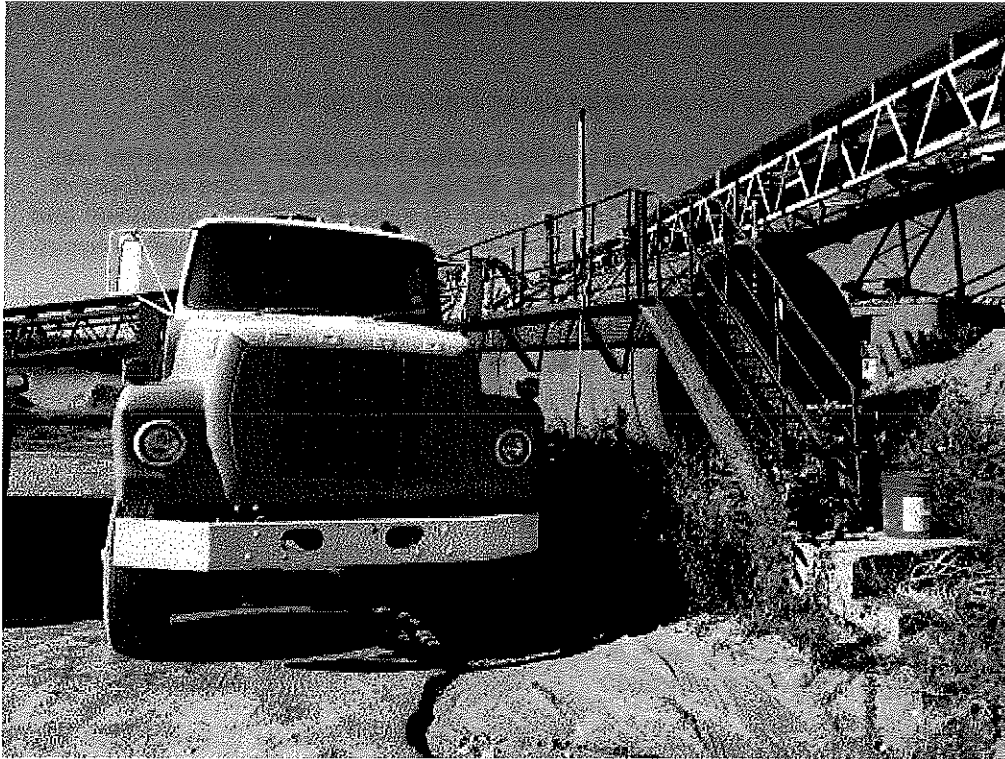
Image 1(014) : Tank and truck for dust suppression.
