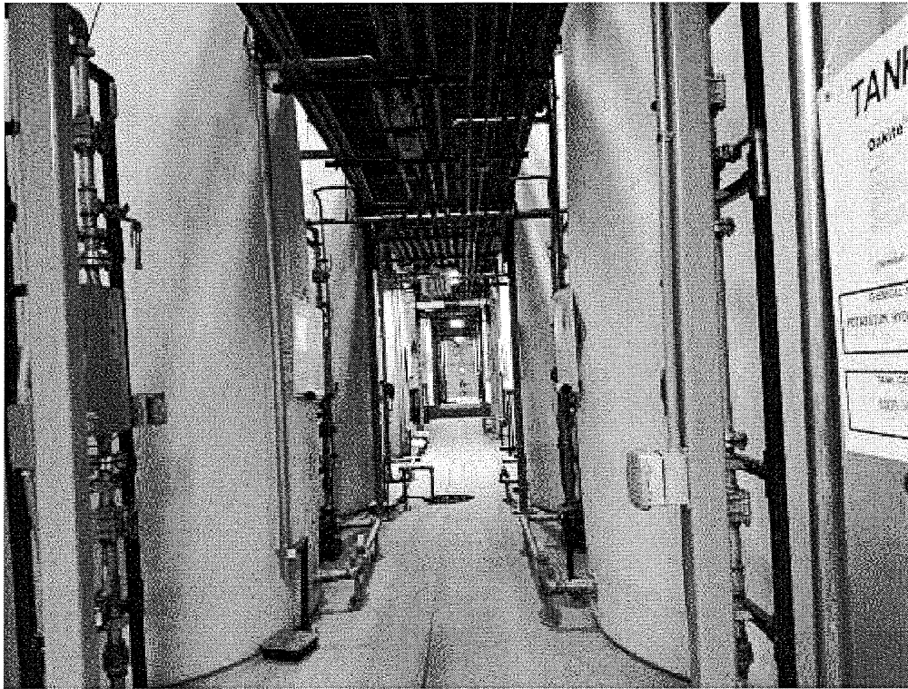
Image 10(Raw Material Area) : Raw Material Storage Area
