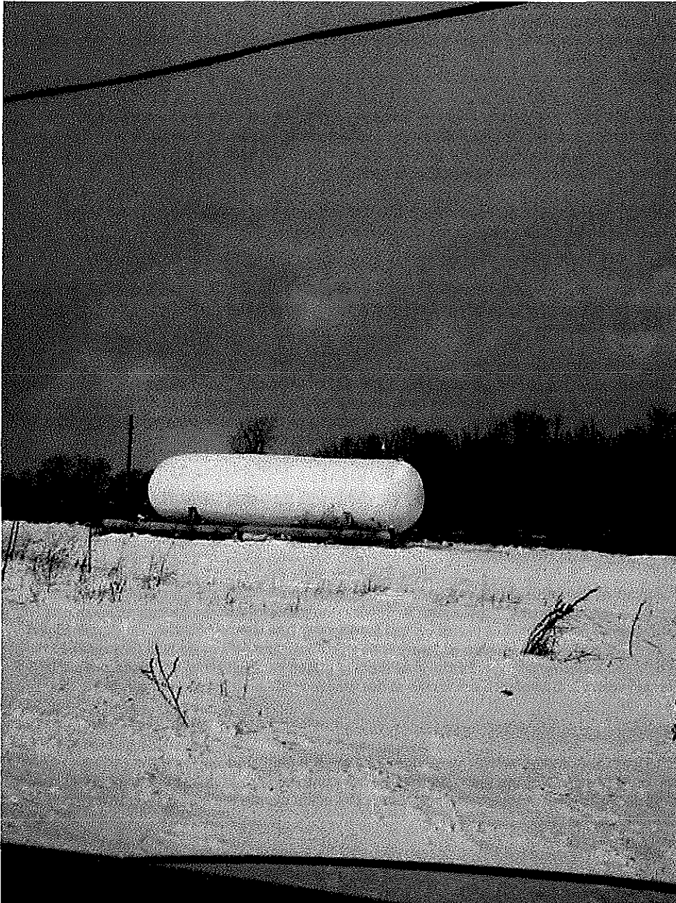
Image 1(NH3 tank) : No stickers present 12/14/16
