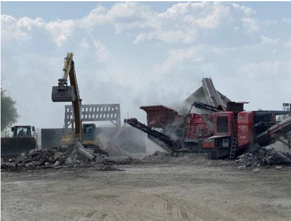
Image 2(2) : Dust from Terex Finlay feeder, primary crusher, and side conveyor, identified as ID # TF, TD, and TDS, respectively, in PTI 69-23.
