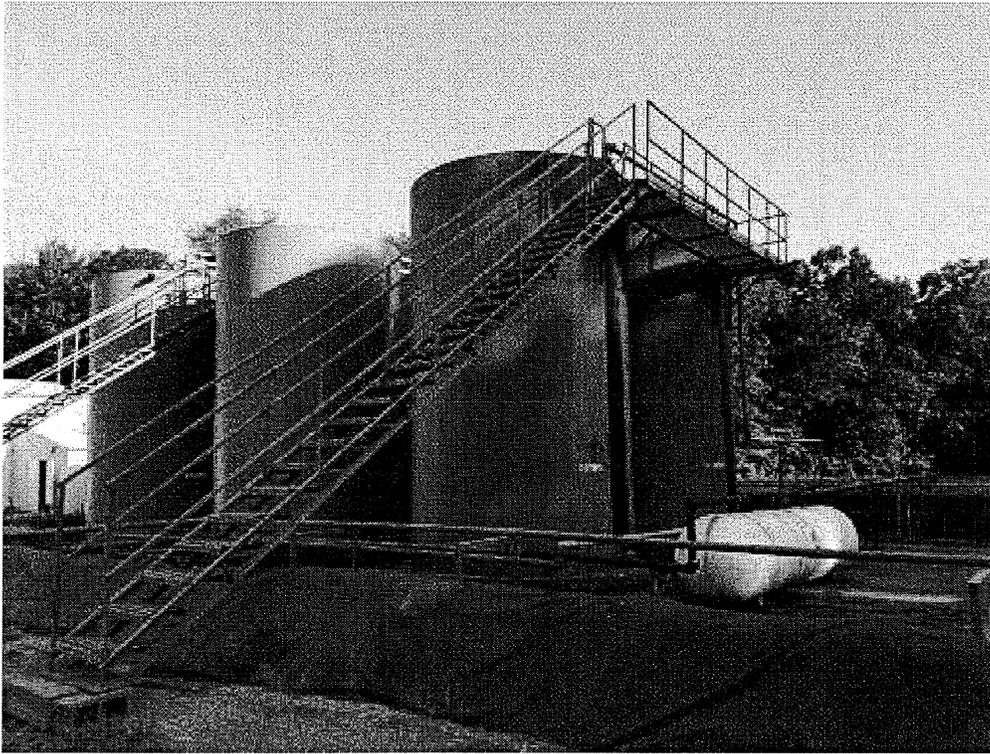
**Image 8(Crude Oil tanks)** : Crude oil tanks. The 2 tanks on the right side are brim tanks. The brim tank in front had a leaky pressure relief hatch.
