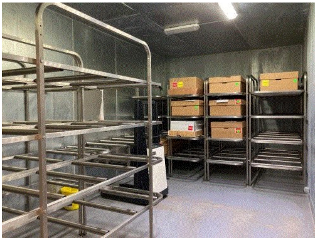
Image 1(IMG 0174.JPG) : Walk-in refrigeration unit with a 24-body capacity. The thermostat is set at 38-39 degrees F.
