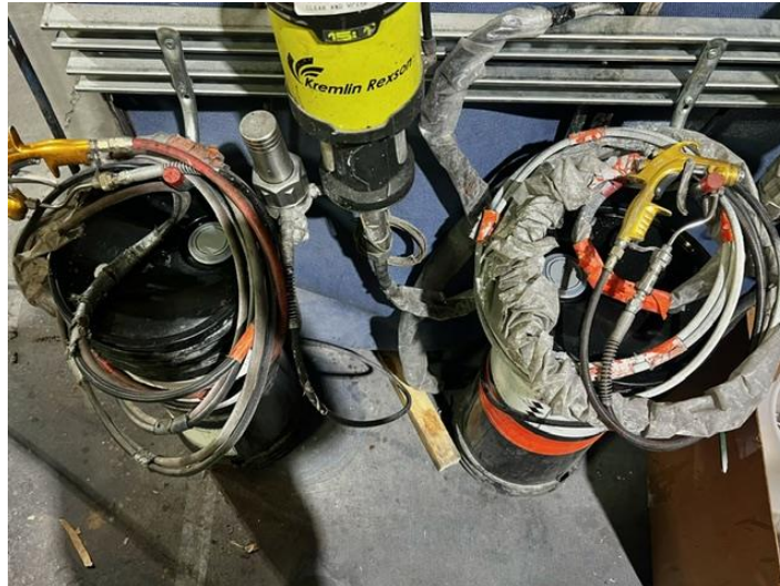
Figure 1: The closed waste container at EU – Spray Booth
