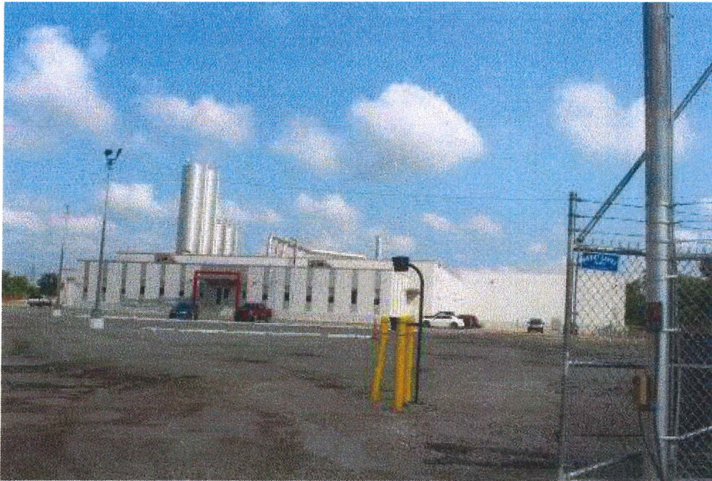
Image 1(VernDale Weaver St) : Front of the VernDale Weaver Street facility.
