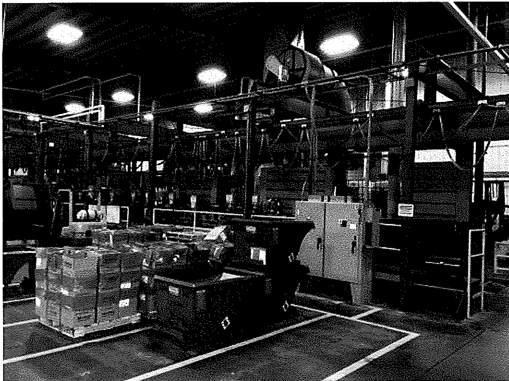
Image 4( Coating Line ) : Coating Line with local ventilation (see slatted gray ducts near bath tanks)
