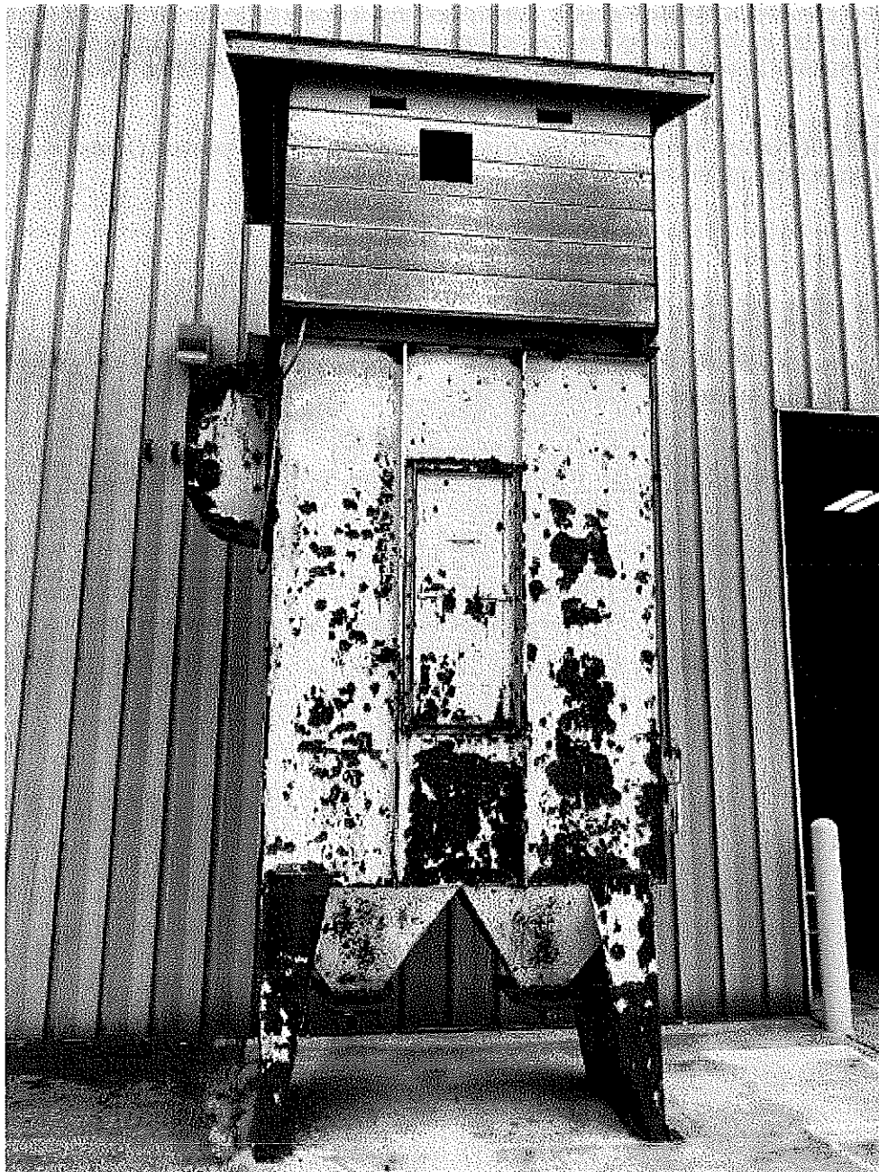
Image 2(cartridge filter #2) : Cartridge filter baghouse unit used for the other 2 shotblasting units
