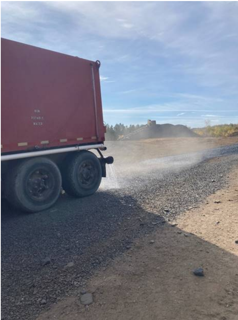
Image 2: Water being applied
