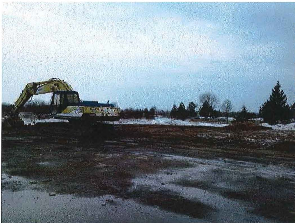
Image 1(fp1) : Cleared and leveled demolition site
