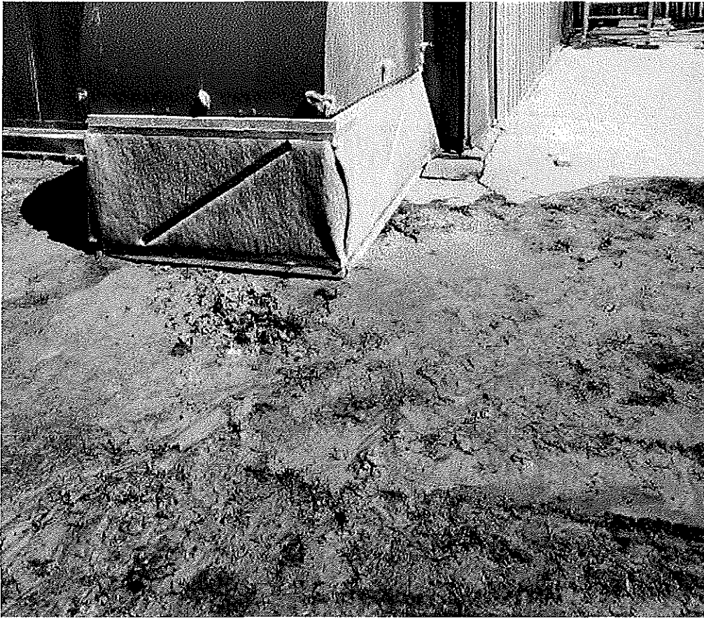
Image 2(Fugitive Dust) : Note blast media on ground (grayish in color).
