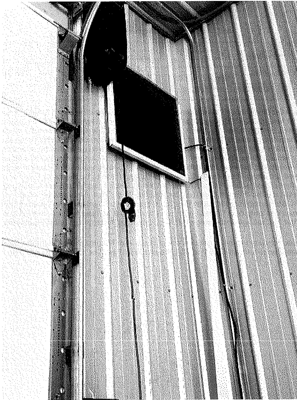
Image 1(Installed filter) : View from inside the building.
