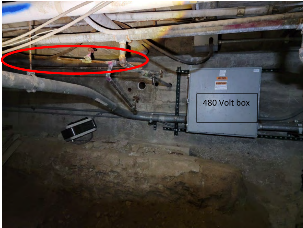
Photo 1 – View of crawl space piping, Copper Line that was abated using glove bag method Note location of 480V Box.
