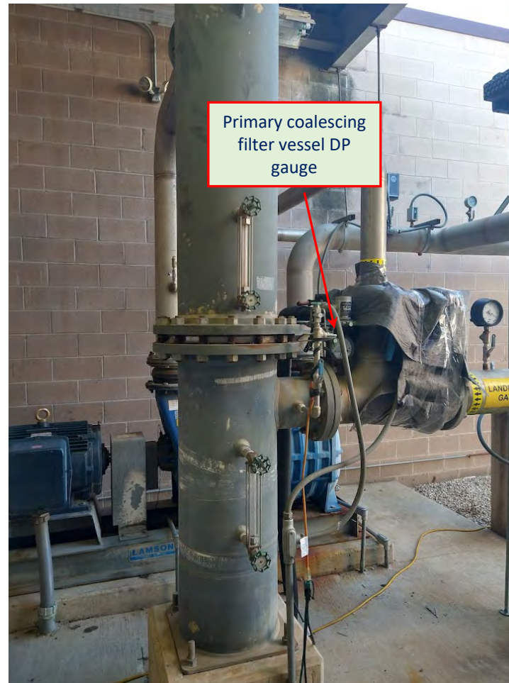
5. Primary coalescing filter vessel DP Gauge
